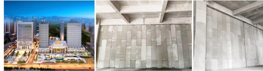
**School cases:** Schools usually have high sound insulation requirements. LESS PANEL are mixed and used in such projects to meet the sound insulation requirements of the projects, while also buying time for other processes and accelerating the construction pace of the project.
