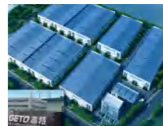
Dingxi Factory 甘肃定西
