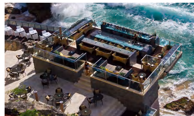
AYANA Resort and Spa Location: Bali, Indonesia Project: Hotel Year: 2007 Product: Multilayer plumbing system
